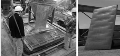
Figure 2. Full-scale formwork and completed concrete panel (C.A.S.T. photos).
