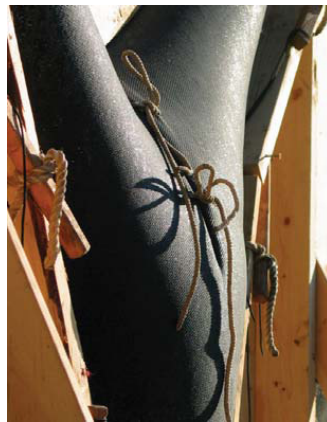
Fig. 2: Photo of a textile formwork.
