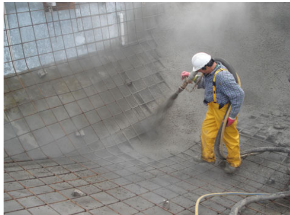
Fig. 3: Photo showing spray applied concrete.
