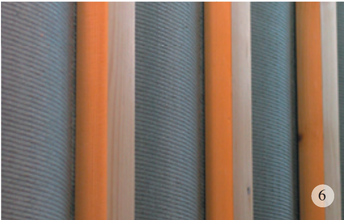
Fig. 6 shows a detail of an interior detail of a URC wall used in a commercial building by architect Shunji Kondo. Unno also acts as a consultant for other architects and builders wishing to use his URC formwork methods
