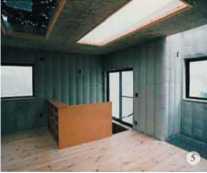
Fig. 5 is an image of the first building 2 constructed with cast-in-place fabric-formed walls. The two skylights shown are experimental passive (evaporative) cooling devices: the one on the right containing water, and the one on the left containing water-soaked charcoal (to increase the rate of evaporation).
