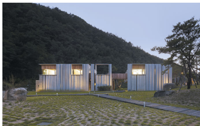
Fig. 20. Hanil Guest House, Seoul, South Korea (2009). Reproduced by permission of Byoung Soo Cho architects, Nicholas Locke
