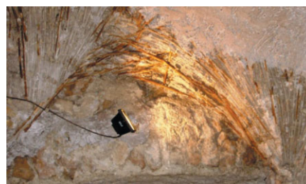
Fig. 2. Reed centring in the Roman concrete vaults beneath the Villa Medici, Rome. Reproduced by permission of Matthew Bronski
