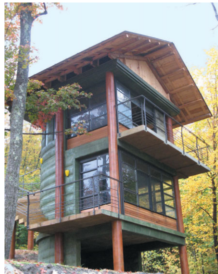
Fig. 15. Black Tree House (2007) during construction of fabric-formed walls and columns, and after completion. Reproduced by permission of Arro Design, Sandy Lawton
