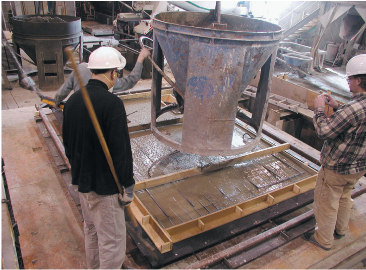
Fig. 14. Wall panel system developed by CAST
