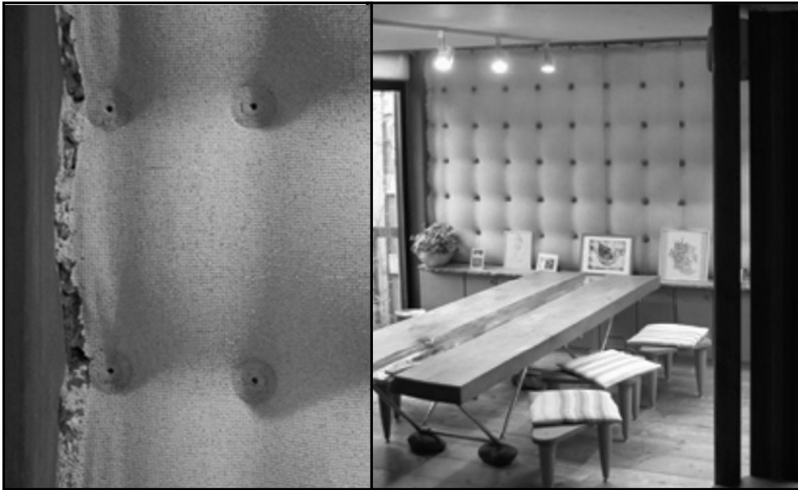
Figure 2. Quilt-like formwork pattern used for the Eiji Hoshino Residence (Mark West photos).
