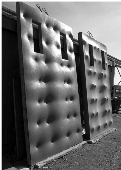
Figure 10. Completed concrete wall panels (C.A.S.T. photo).
