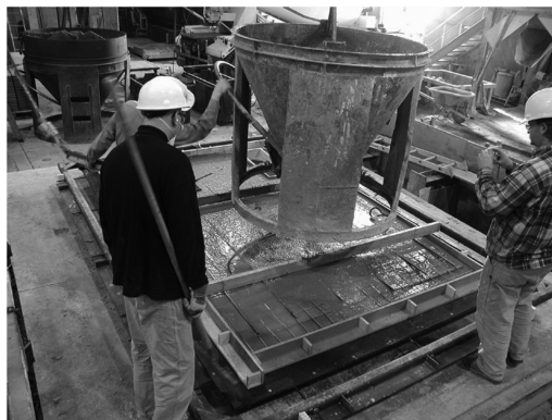
Figure 9. Placing concrete in full-scale wall panel formwork (C.A.S.T. photo).
