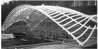
5-1: Linear support in a free form formwork [b]
