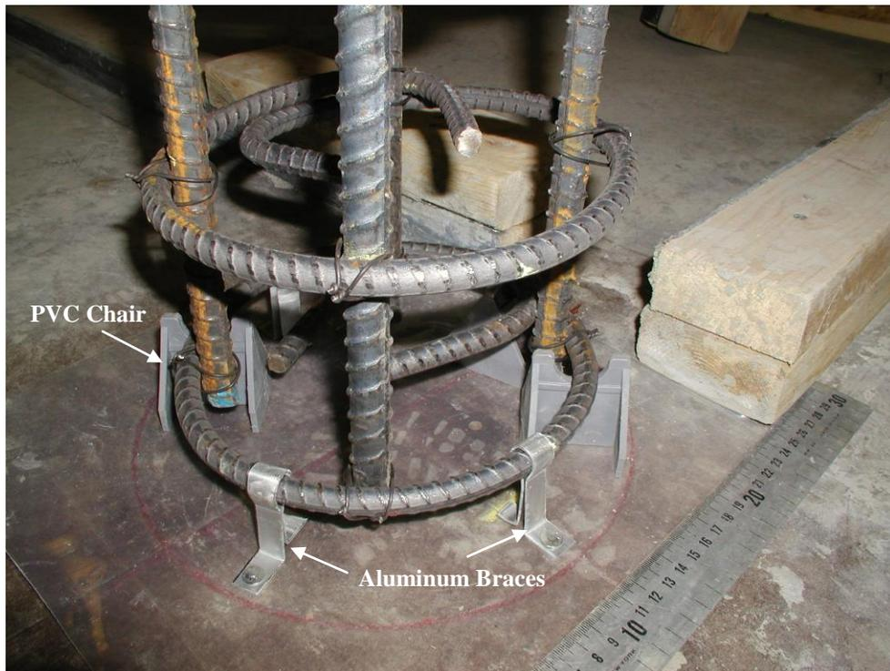
Figure 45: Details of the bottom of the column
