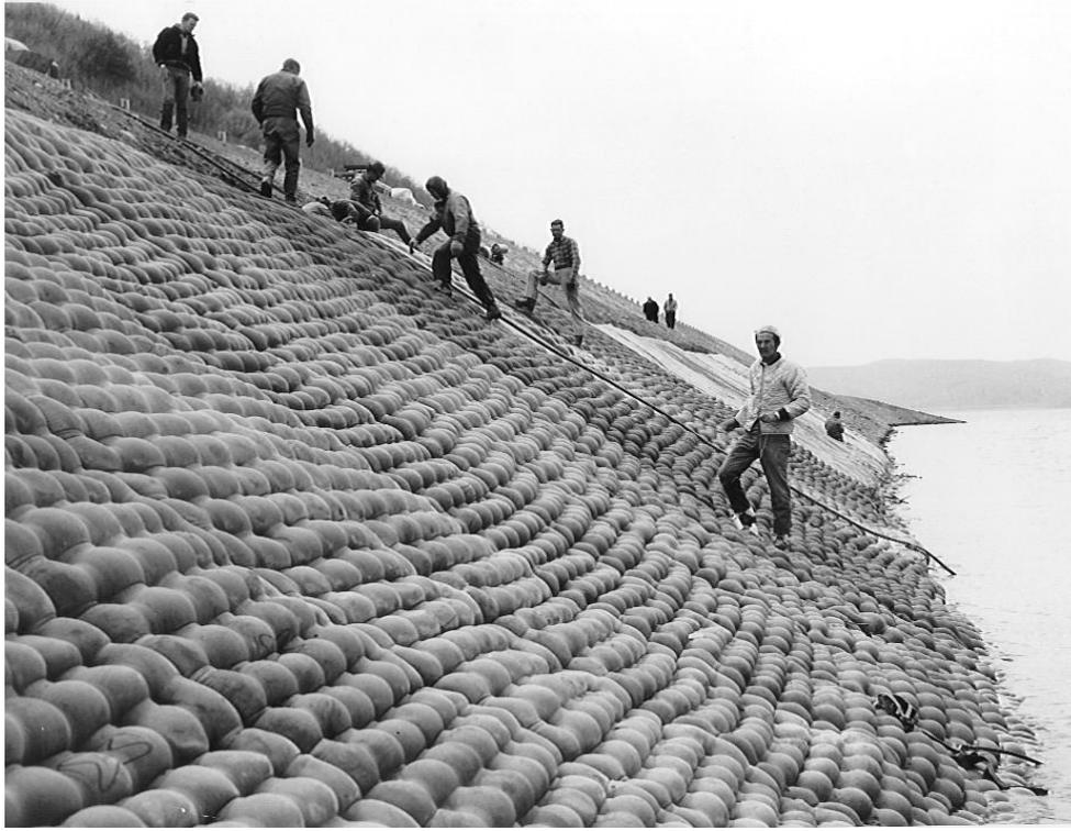
**Figure 5: River bank stabilization bags (Fabriform) installed in 1967 on the Allegheny Reservoir, New York ([www.fabriform1.com](http://www.fabriform1.com) 2009)**
