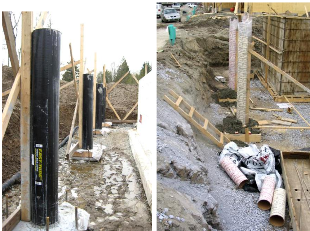
Figure A1: Commercially available column fabric formwork called Fast-Tube™ (left) and conventional cardboard formworks (right) on a job site
