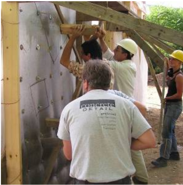
"Vibrating" Concrete
