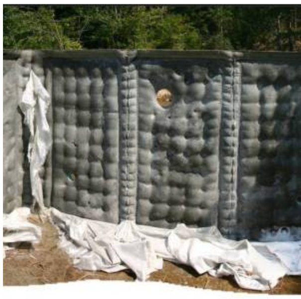
Stripping Formwork
