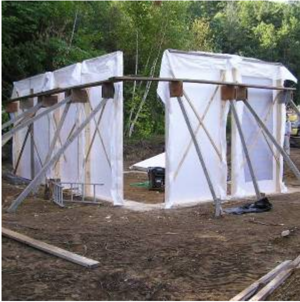
Wall Form Placement
