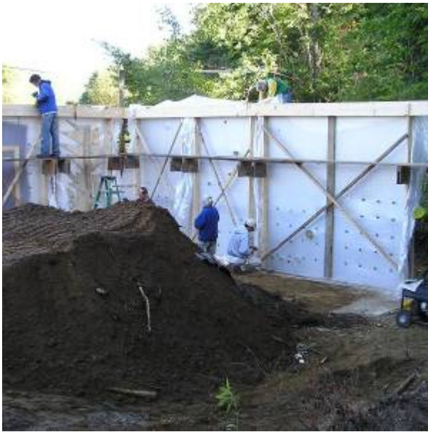
Wall Form Placement
