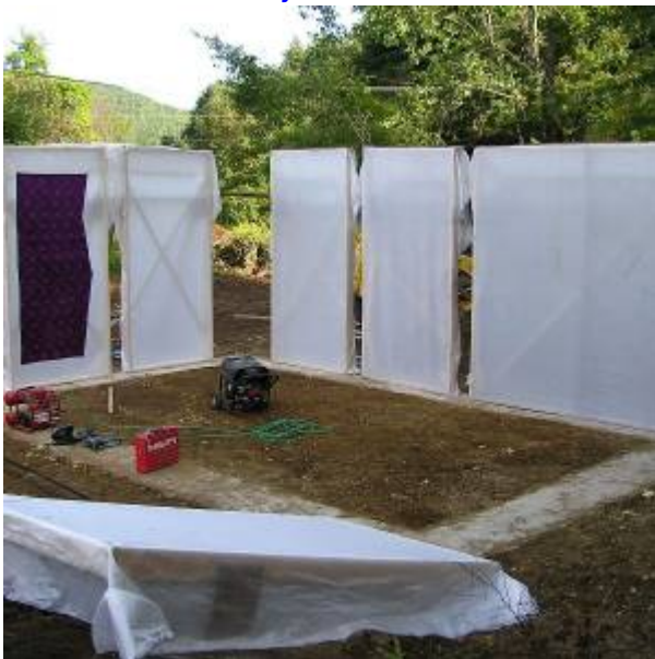
Wall Form Placement
