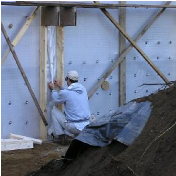
Wall Form Placement
