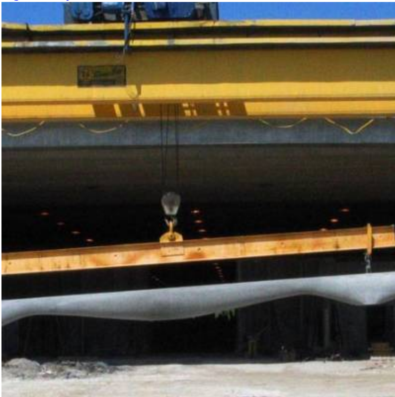
Fig. 12. Completed full scale variable section concrete beam.
