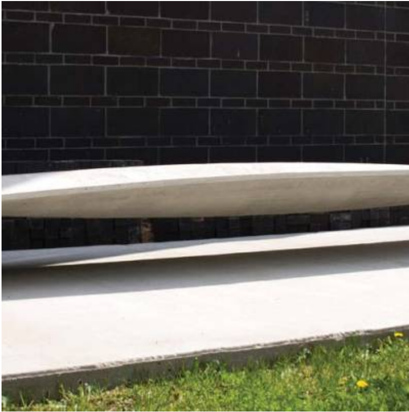
Fig. 41. Completed double-curvature lenticular thin-shell vault.
