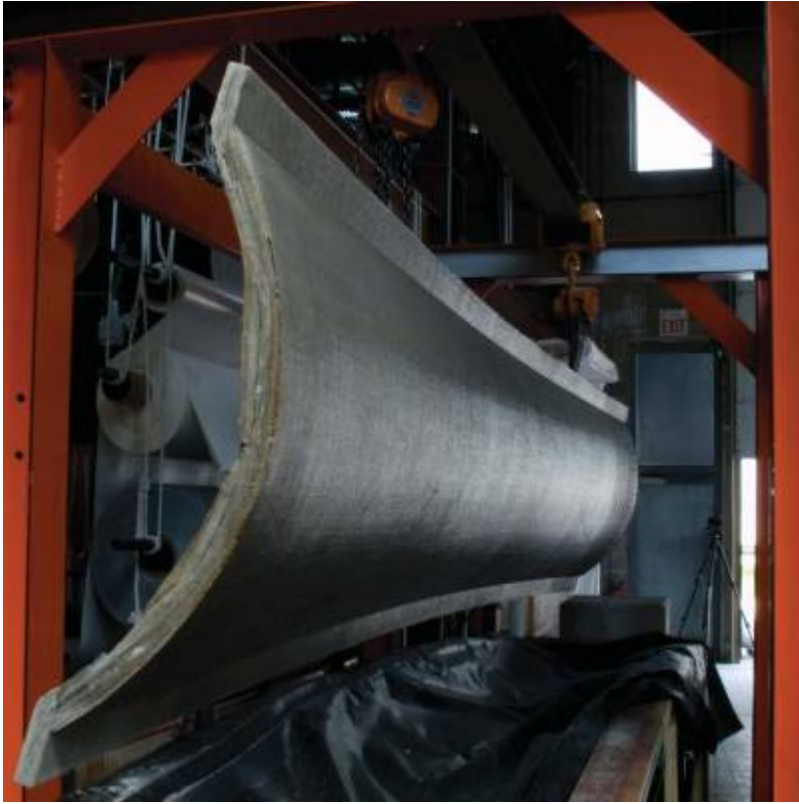
Fig. 35. Removing 3 cm (1.2 in) vault from formwork.
