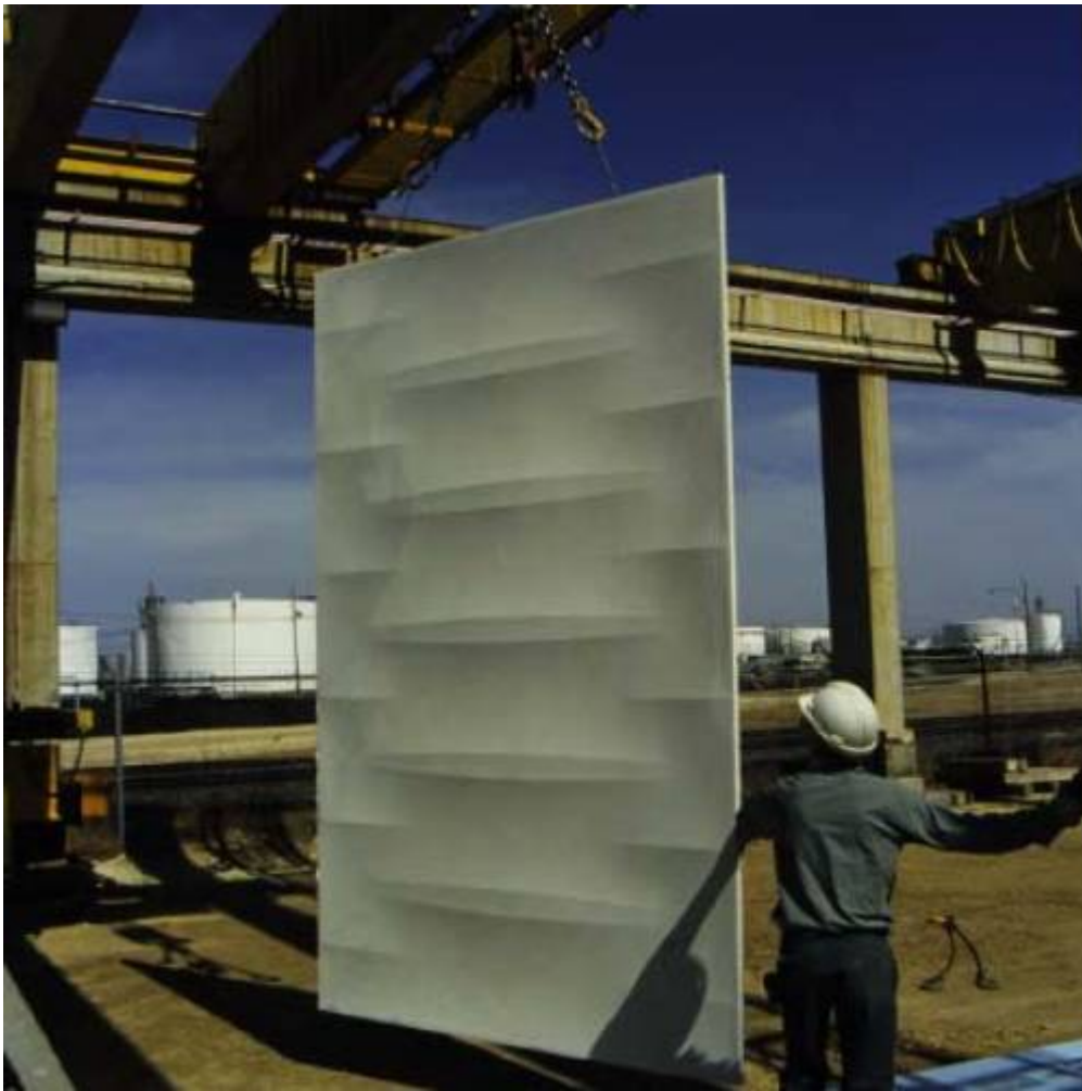
Fig. 11. Completed full scale reverse cast GFRP panel.
