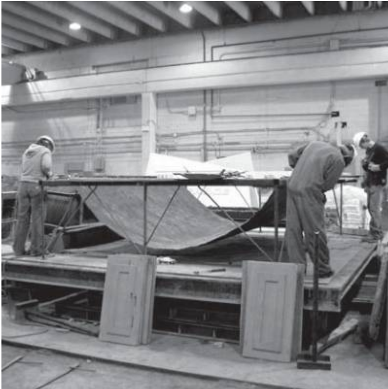
Fig. 22. Step 1 - Geotextile fabric hung from a frame.
