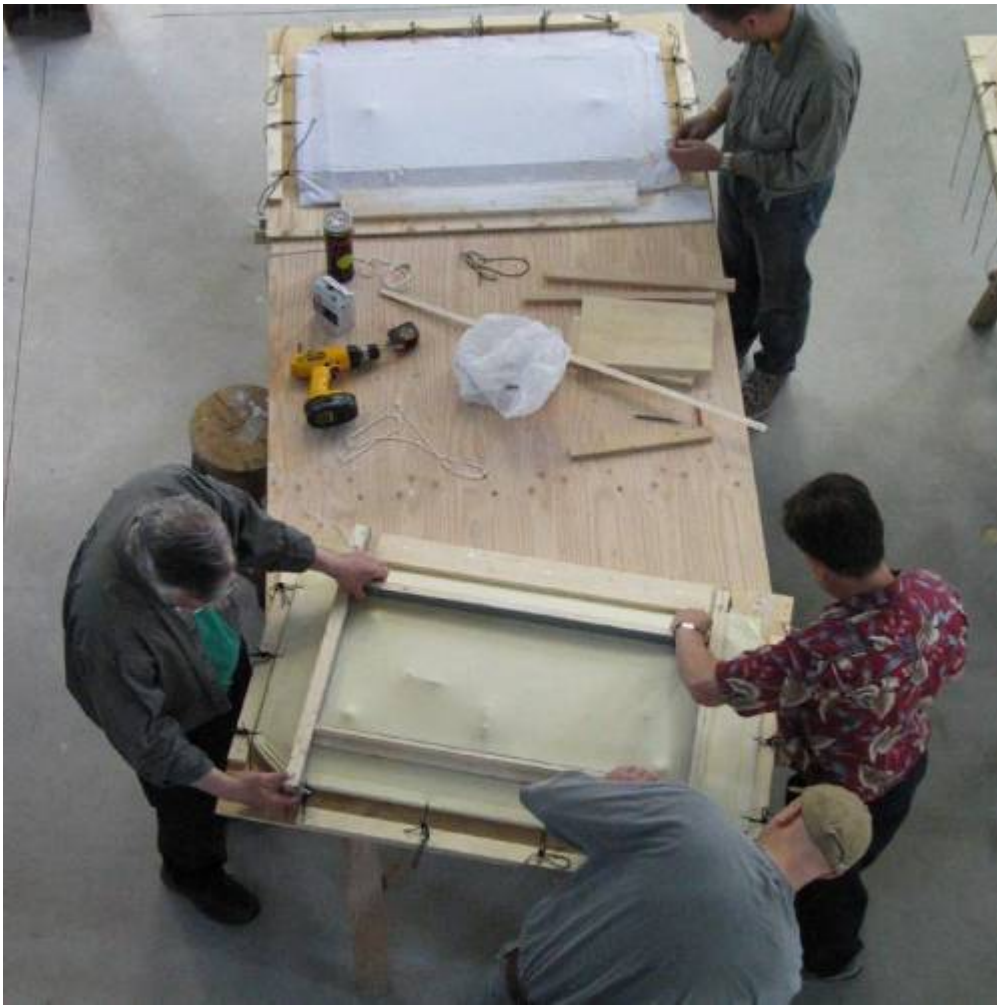
Fig. 2. Model wall panel formwork.
