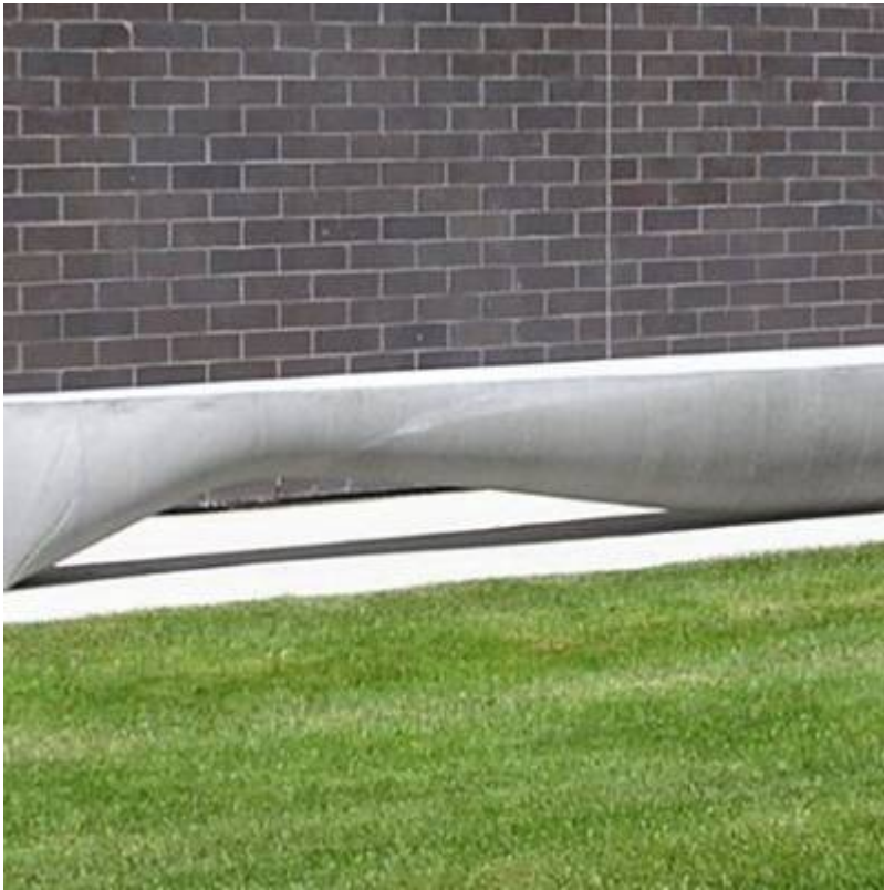
Fig. 13. Concrete beam installed at C.A.S.T.
