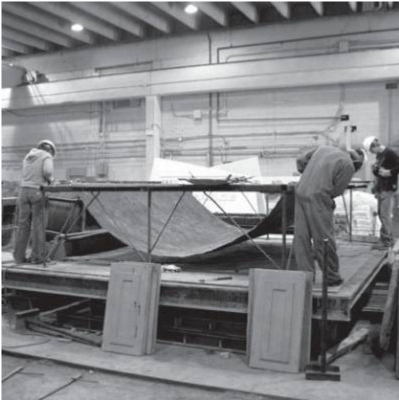
Fig. 22. Step 1 - Geotextile fabric hung from a frame.
