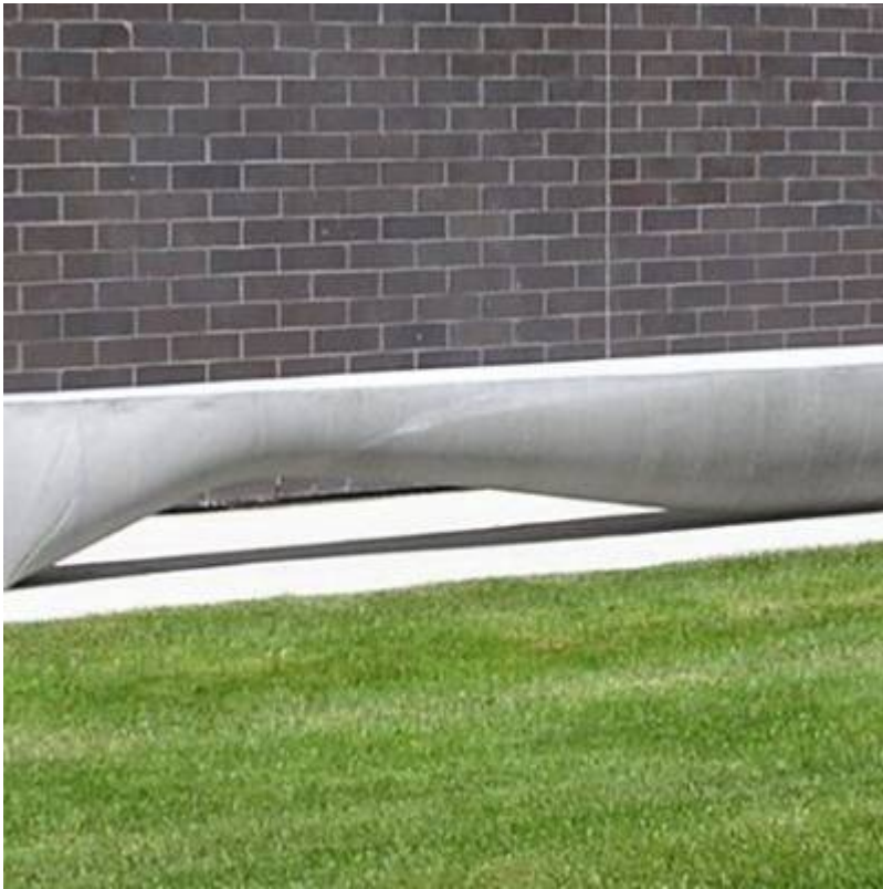
Fig. 13. Concrete beam installed at C.A.S.T.
