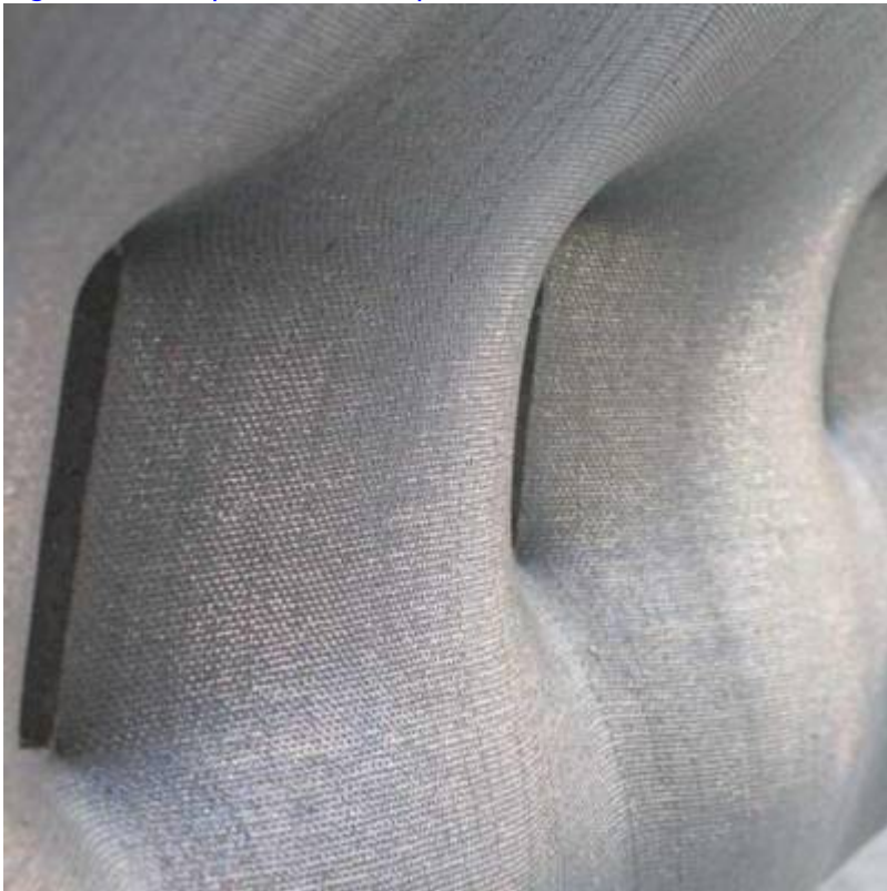
Fig. 10. Close up view of variable section concrete 'pinch' beam finish.
