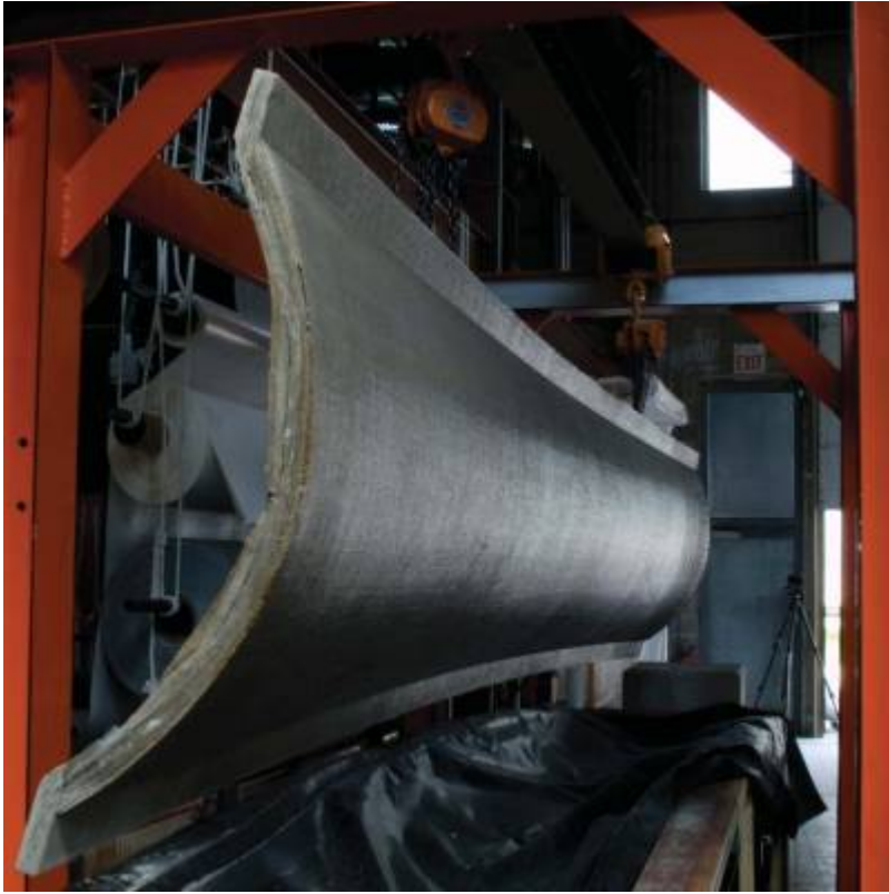
Fig. 35. Removing 3 cm (1.2 in) vault from formwork.
