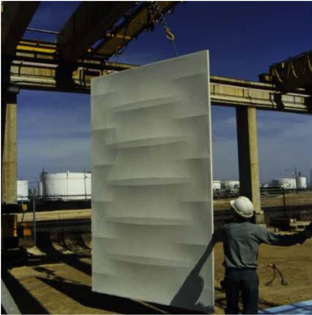
Fig. 11. Completed full scale reverse cast GFRP panel.
