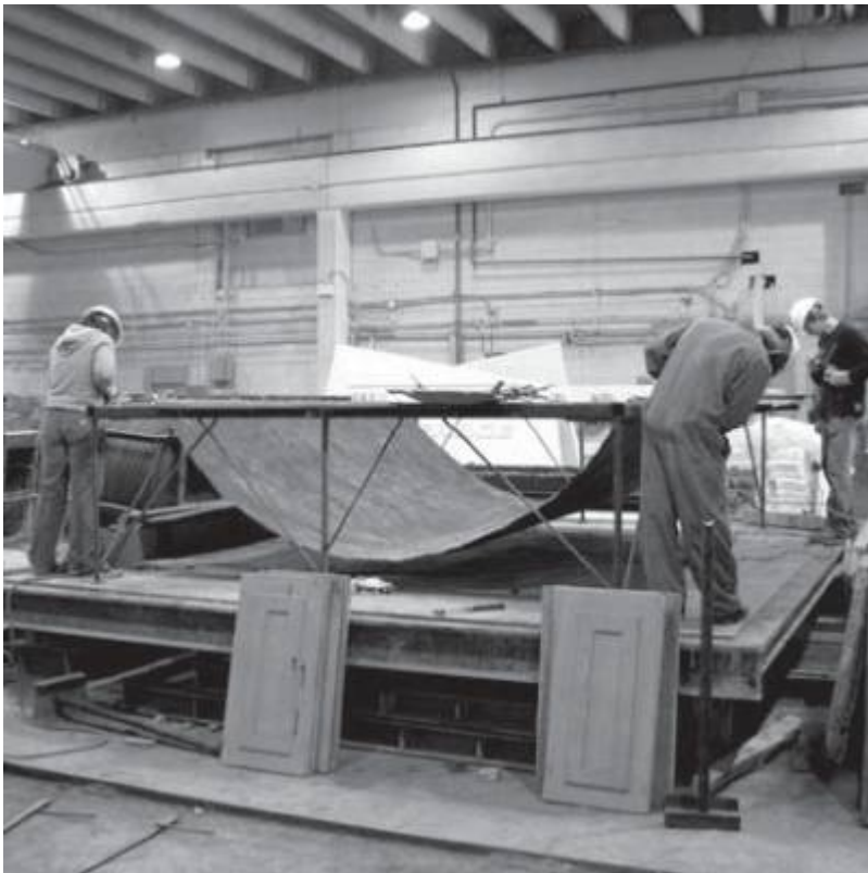
Fig. 22. Step 1 - Geotextile fabric hung from a frame.
