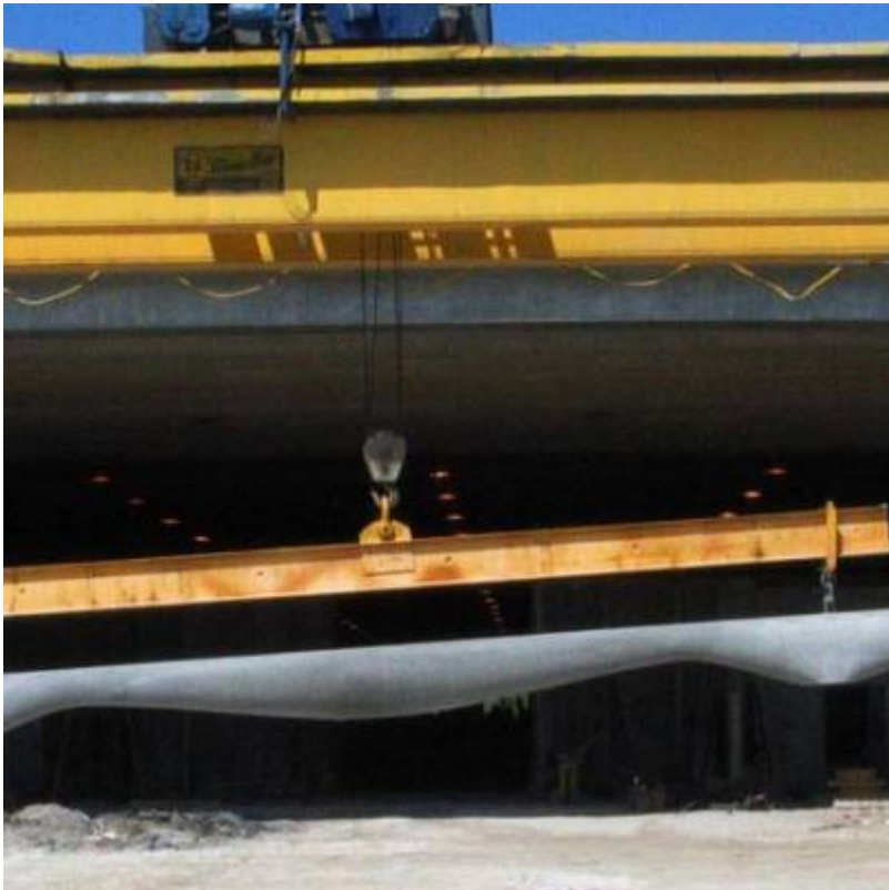
Fig. 12. Completed full scale variable section concrete beam.
