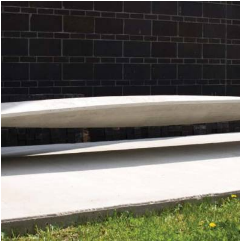
Fig. 41. Completed double-curvature lenticular thin-shell vault.
