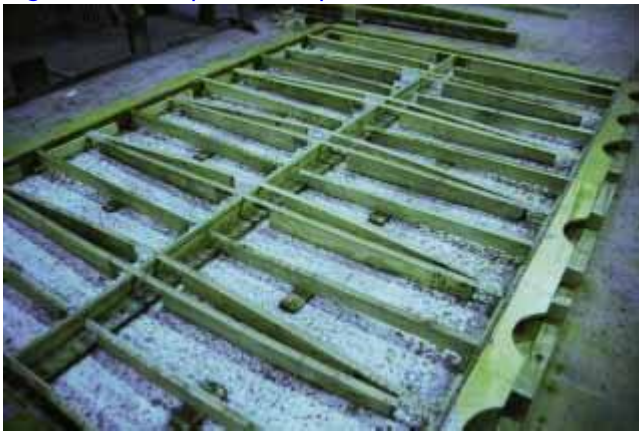
Fig. 9. Formwork for full scale wall panel.
