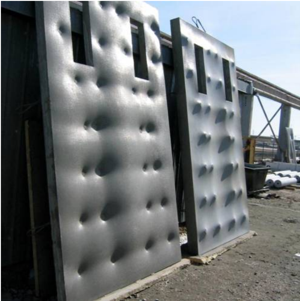
Fig. 7. Completed concrete wall panels.
