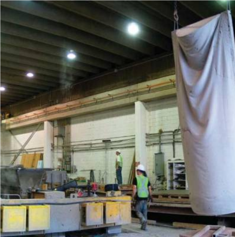
Fig. 46. Thin-shell panel cast from a sheet of hanging geotextile fabric used as...
