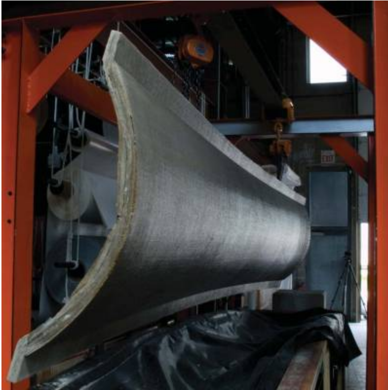
Fig. 35. Removing 3 cm (1.2 in) vault from formwork.
