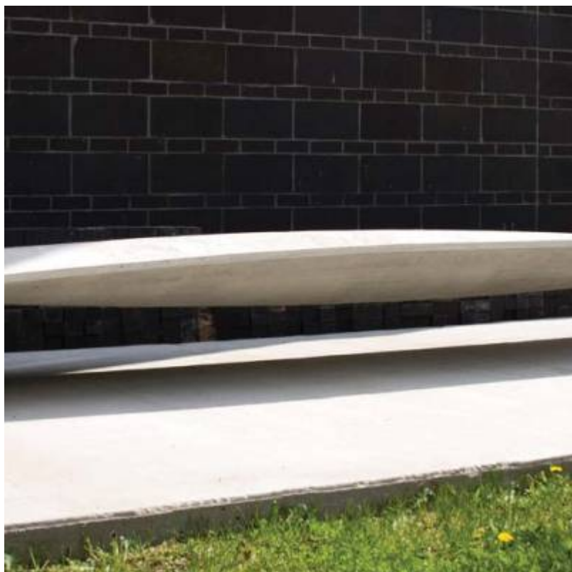
Fig. 41. Completed double-curvature lenticular thin-shell vault.
