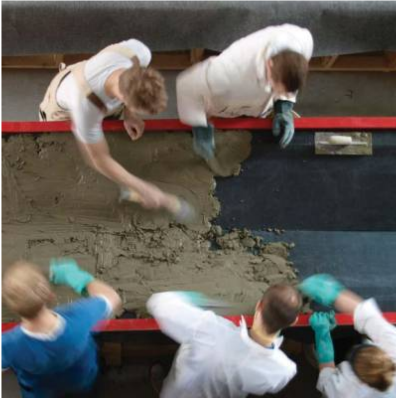
Fig. 39. Placing concrete and carbon grid (Portland cement mortar mix used) for...
