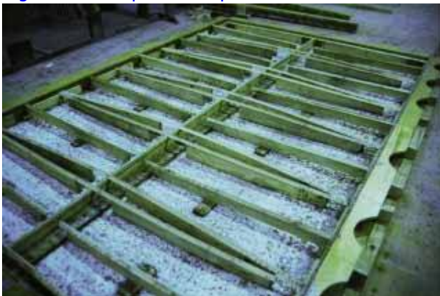
Fig. 9. Formwork for full scale wall panel.
