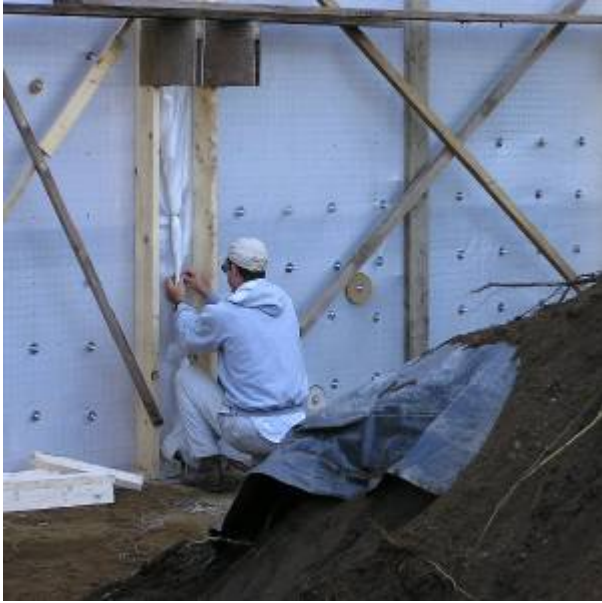
Fig. 7. Wall Form Placement
