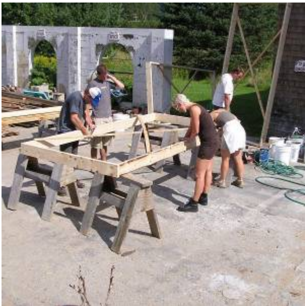
Fig. 1. Wall Form Assembly
