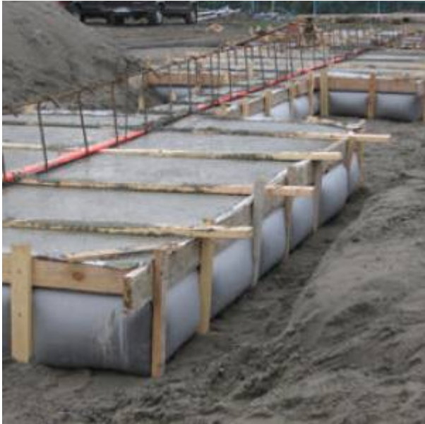
Fig. 2. Spread/Continuous Footing Application
