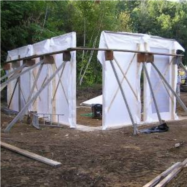
Fig. 5. Wall Form Placement
