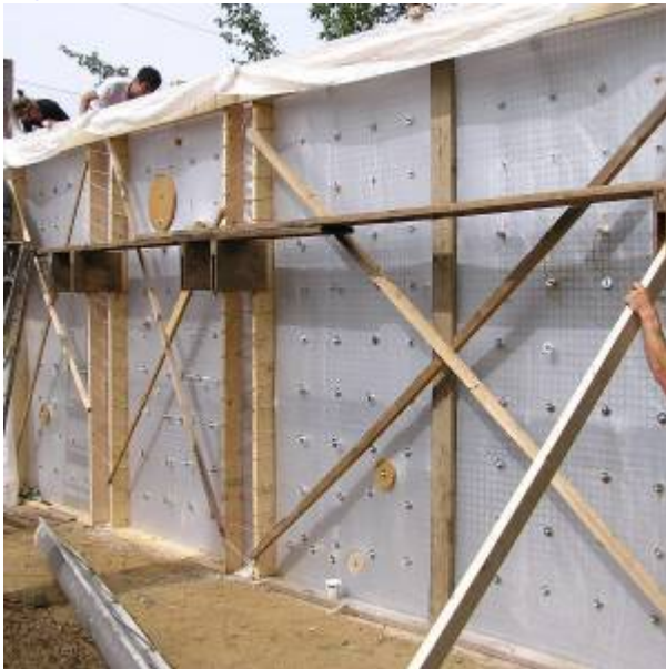
Fig. 8. Wall Form Placement
