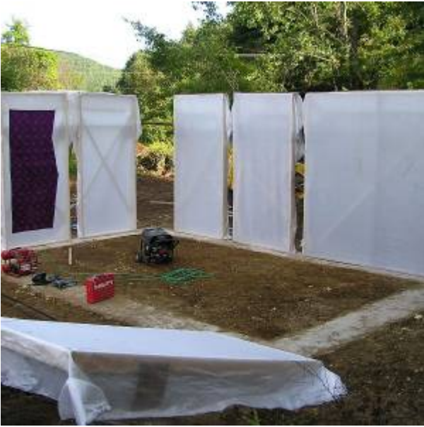
Fig. 4. Wall Form Placement
