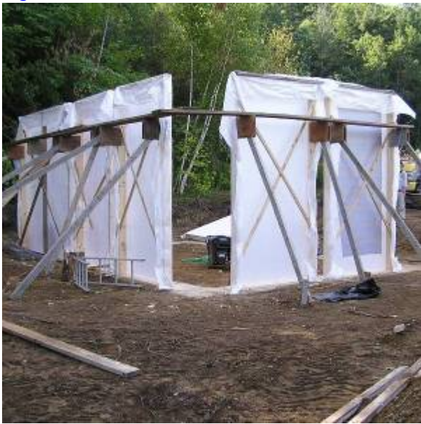
Fig. 5. Wall Form Placement
