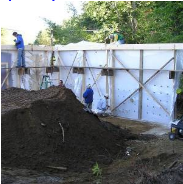
Fig. 7. Wall Form Placement
