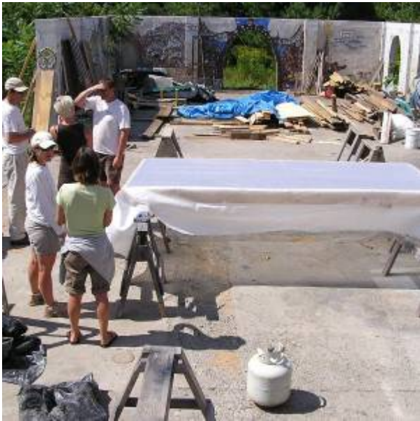
Fig. 2. Wall Form Assembly
