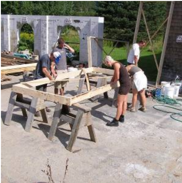
Fig. 1. Wall Form Assembly
