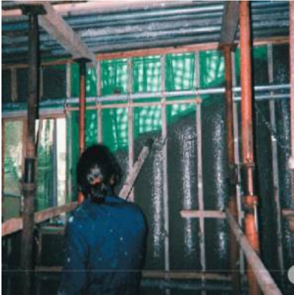
Fig. 1. Frame Form Method
