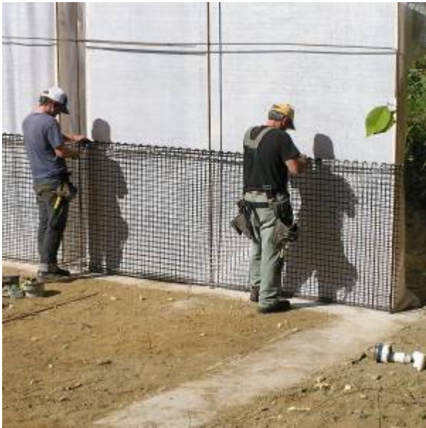
Fig. 6. Adding Carbon Fiber Grid
