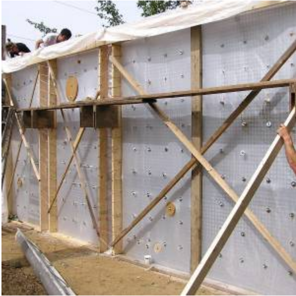
Fig. 8. Wall Form Placement
