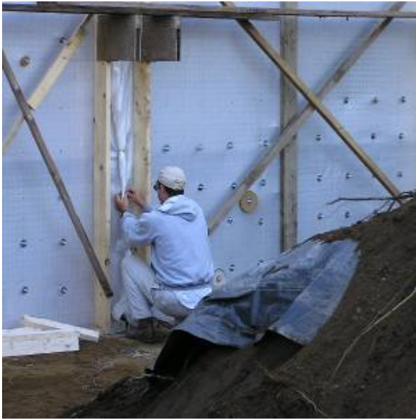
Fig. 7. Wall Form Placement
