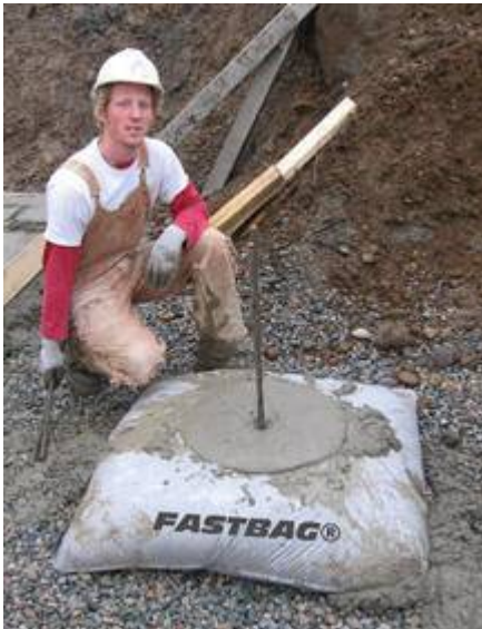
Fig. 3. Spread Footing Application
