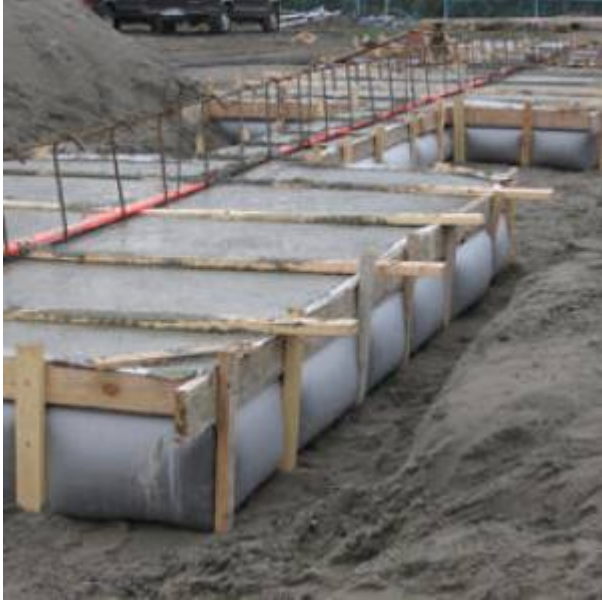
Fig. 2. Spread/Continuous Footing Application
