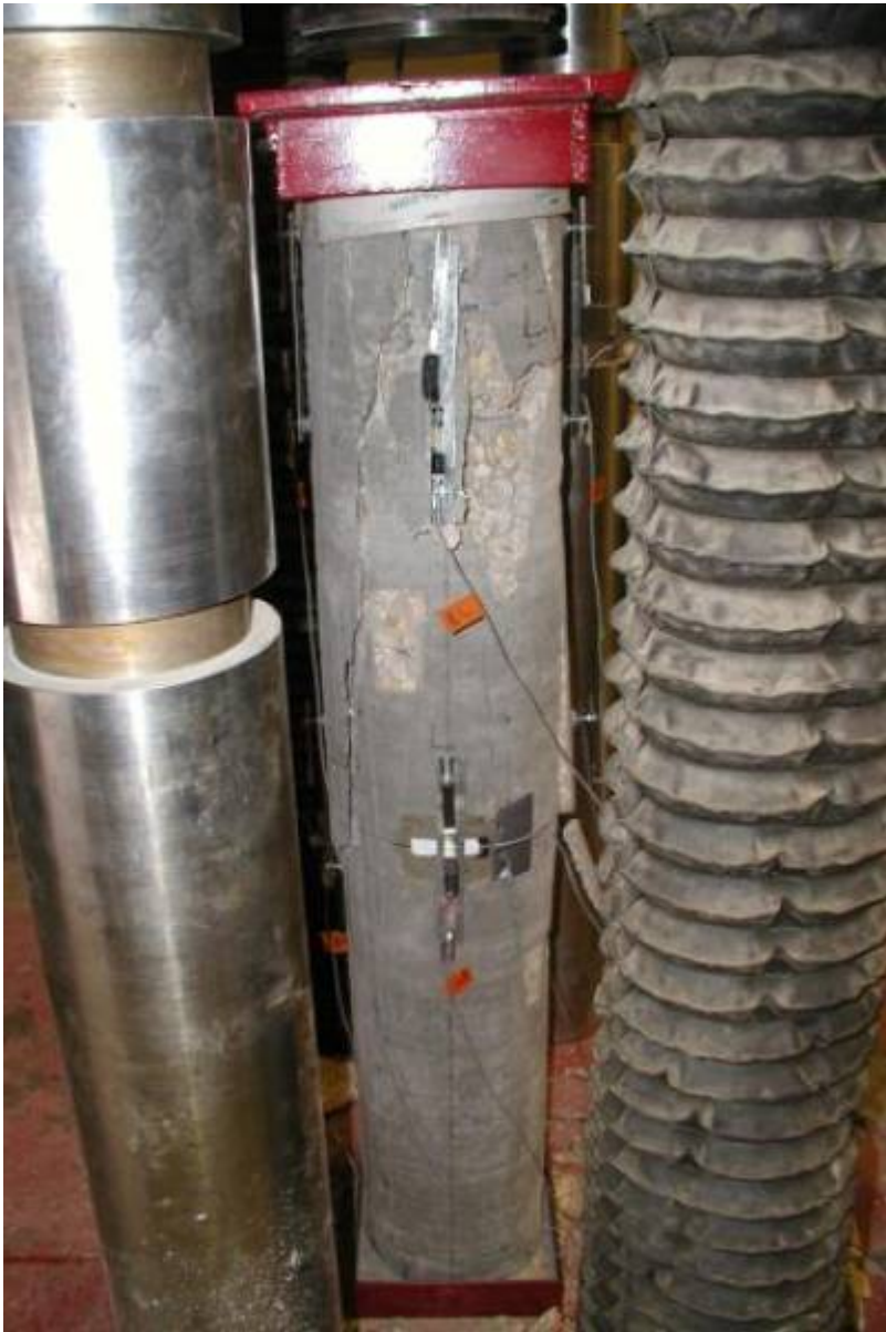
Figure 65: Column FF-FAC after failure.
