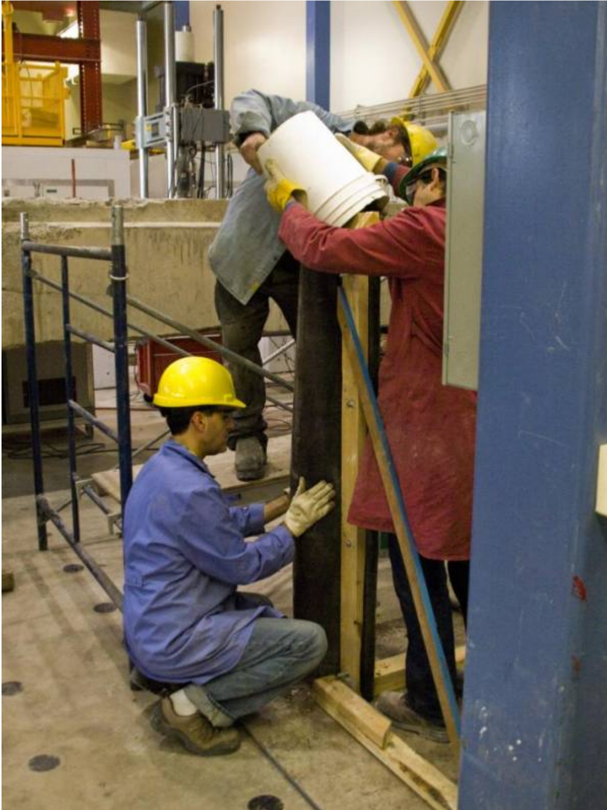
Figure 47: casting of column in fabric formwork.
