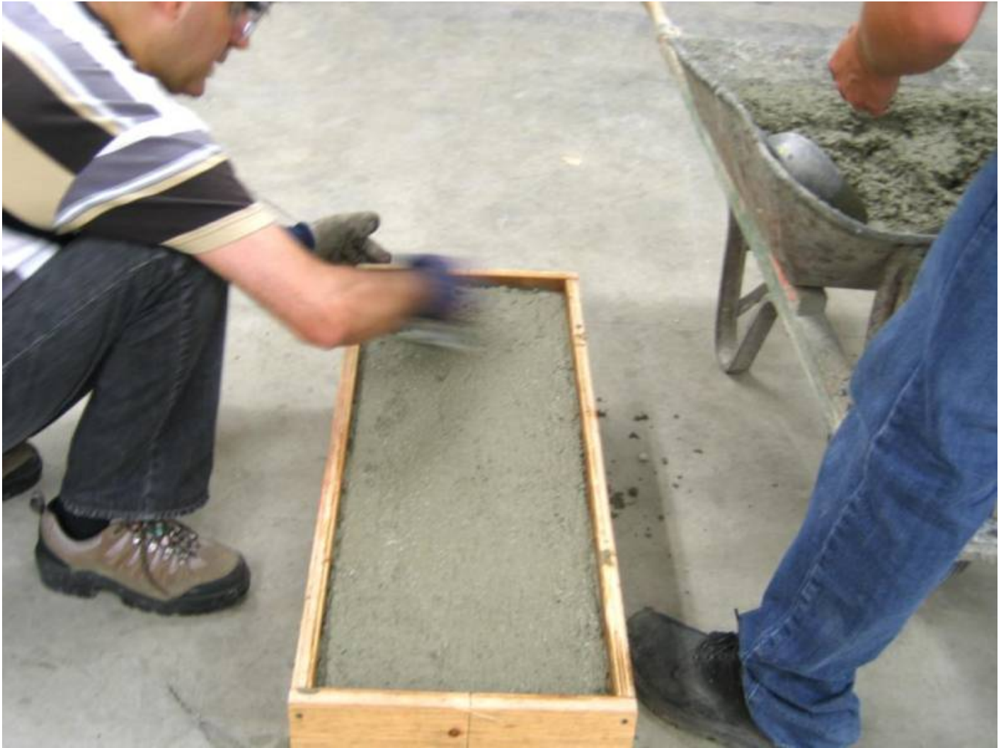
Figure 9: Filling the box with fresh concrete.
