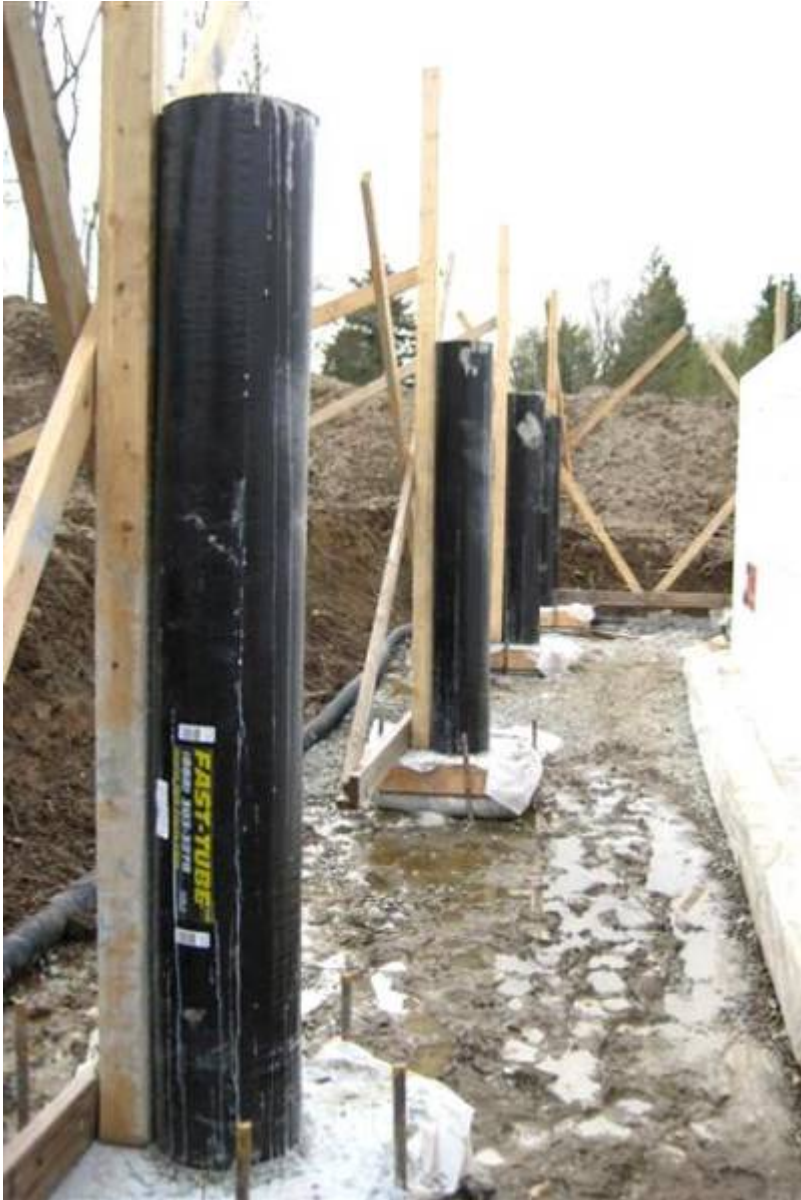
Figure A1a: Commercially available column fabric formwork called Fast-Tube™ on...
